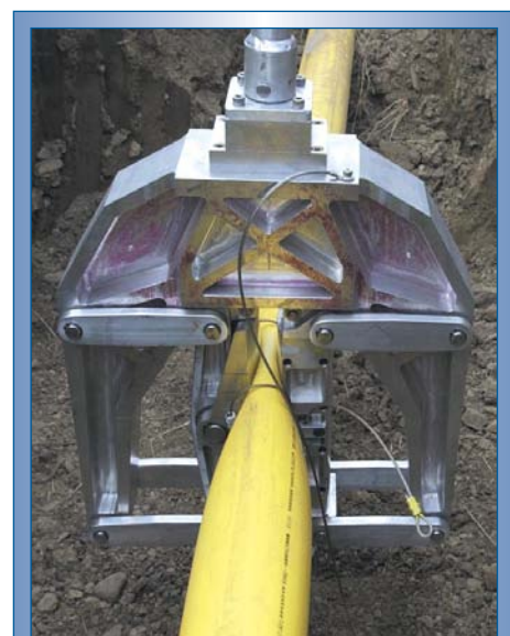
Figure 14. Pipe integrity maintained following squeezed-off on 6-in. MDPE pipe with the Timberline TR650.
