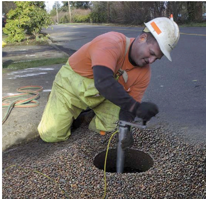
Figure 1: Keyhole excavation
