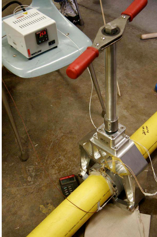
Figure 14: The test tool in the process of applying a repair patch
