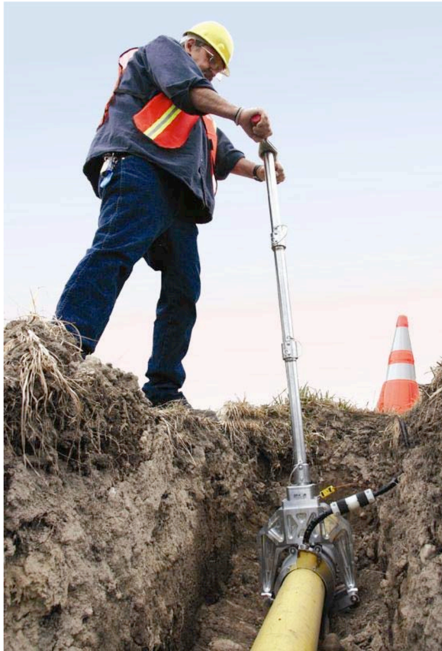
Figure 52: Final engineer prototype applying a PE gel film patch on 4-inch MDPE pipe
