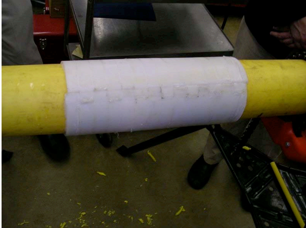
Figure 50: PE gel film patch successfully repaired a damaged 4-inch MDPE pipe
